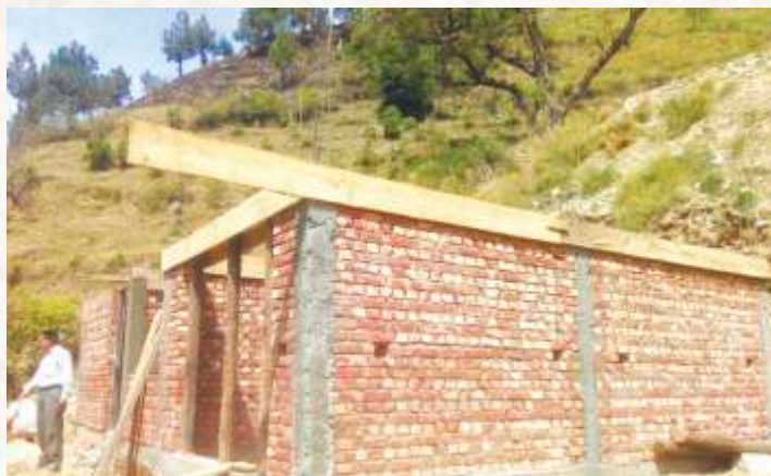
The collection center, Manpur, under construction
